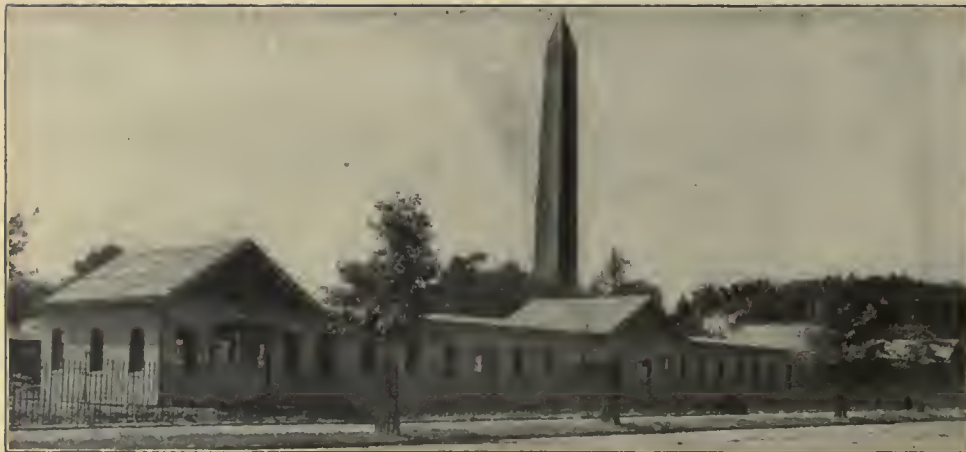
PAROID covers the Plant Industry Buildings, U. S. Department of Agriculture, Washington, D. C
