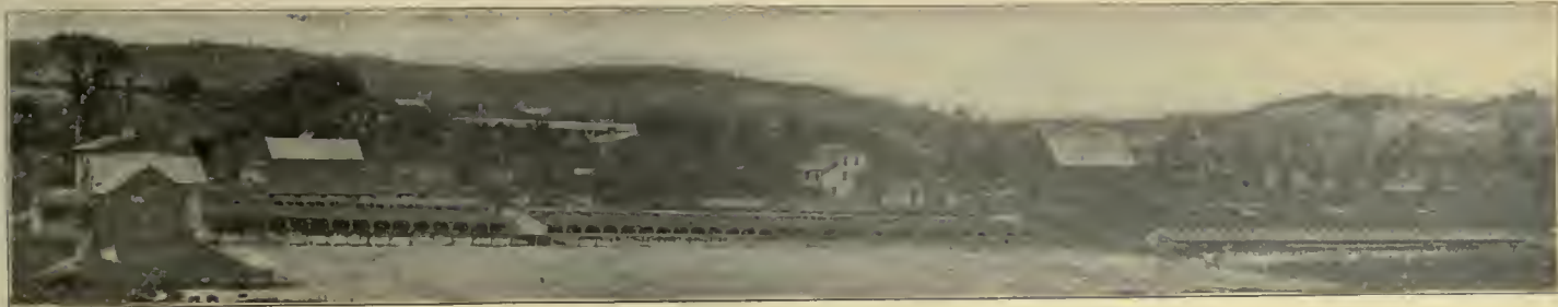
Meadow Brook Farm poultry plant, Dallas, Pa. Roofs are covered with PAROID.
