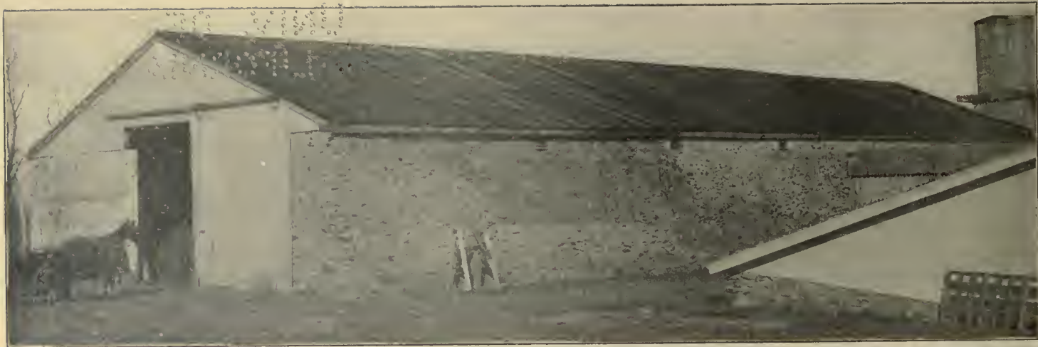
A cow barn, East Greenwich, R. I. Roof covered with PAROID.
