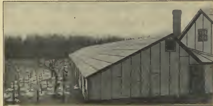
Duck breeding house, roof and sides covered with PAROID, Weber Bros., Pondville Mass.
