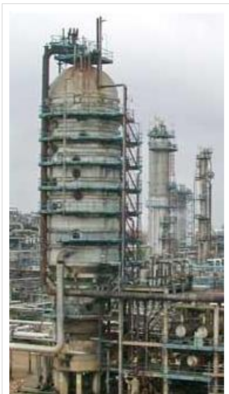
Large-scale, industrial vacuum distillation column [15]
